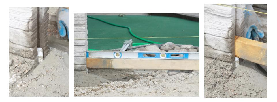
Bottom panel should not touch the earth. Leave a  $\frac{1}{2}$ " to 1" gap between bottom of panel and grade. NOTE: Small diameter PVC pipe is commonly cast in piers to level panels. It is acceptable to bear the concrete panels on the PVC levelers. PVC levelers must be schedule 40 w/a minimum nominal diameter of 1".
