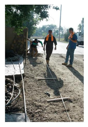
Dig post holes. To determine the proper pier size, reference the pier depth and diameter schedule that is shown on the fence specification drawings, https://signaturestone.com/columns-fencespecifications/ Using a post-holer, dig holes at least 2 feet deep with a diameter of 18". Make sure you follow the rules stipulated in your permit, as many cities have rule regarding hole depth. Remember to call the Digline at 811 before you dig!
