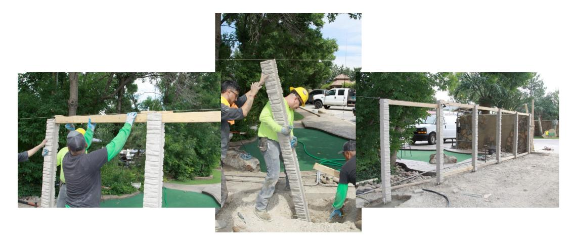
You will want to continue to use string to make sure the posts are in line with each other. Continue setting posts. Get in all the posts before moving on. Use temporary cross bracing to hold posts in place while the concrete hardens. This will take at least 24 hours.
