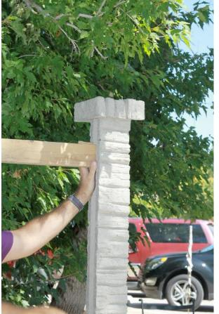
Once the top panel is in the panel caps and post caps are bonded into place by applying Sikaflex-1A adhesive between the cap and fence component.
