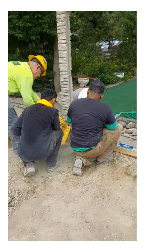
Pour in the concrete, mix with water according to the manufacturer's instructions for a 3,000PSI mix, and continue to use the level as it sets to be sure that it stays straight. Alternatively, mix the quick-set concrete in a bucket or wheelbarrow and then pour it in.
