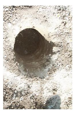
Place posts. Place the 5x5 posts at your preferred height (factoring in the depth of the hole) and place them one at a time. This may require a helping hand. Pour in quick-set concrete. Before setting the concrete, use a post level to ensure that the post is plumb and double check the height to make sure it's what you want.
