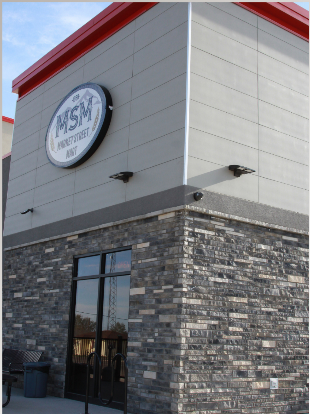
PICTURED: LEDGESTONE CRESTONE MORTAR JOINT INSTALLATION
